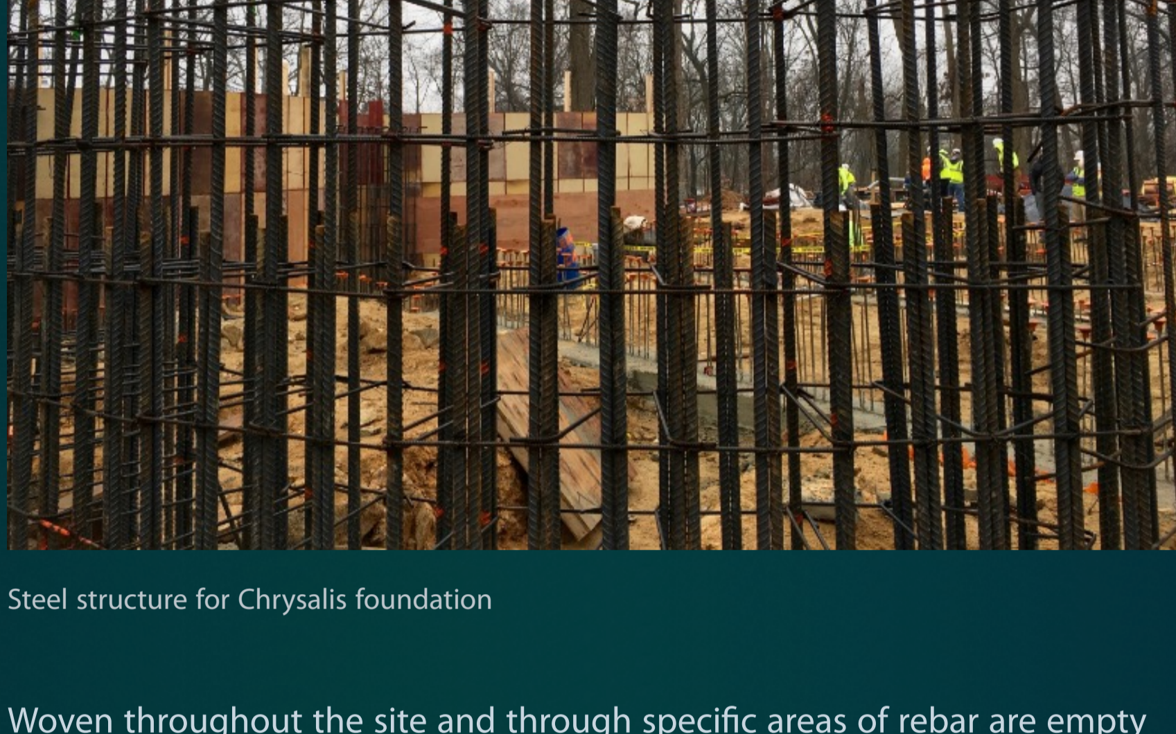
Steel structure for Chrysalis foundation
