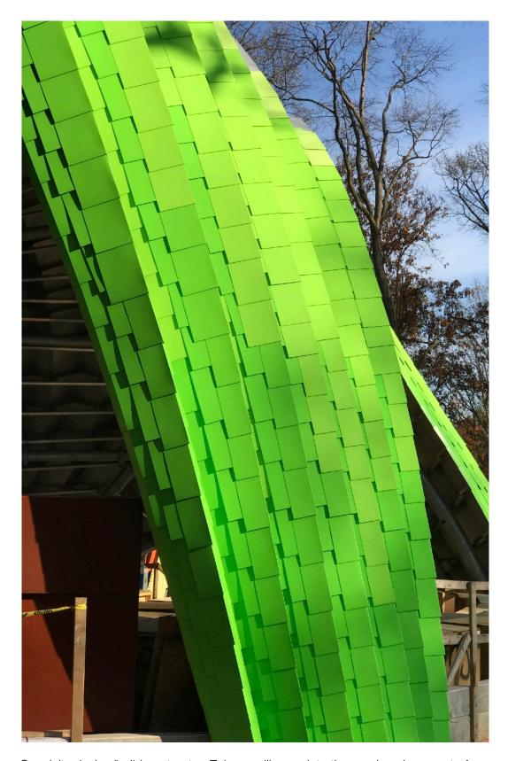
Specialty design/build contractor, <u>Zahner</u>, will complete the precise placement of the 7,700 shingles, with their 45,000 stainless steel rivets, eleven (11) sizes and four (4) <u>Spring Green colors</u>, in December.
